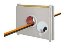
5. Seal the plugs completely at a depth of ≥ 2 mm (dry film thickness ≥ 1 mm) with FLAMMOTECT-A or BMK.
